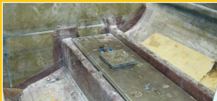
A fuel tank nestled between two bottom girders
