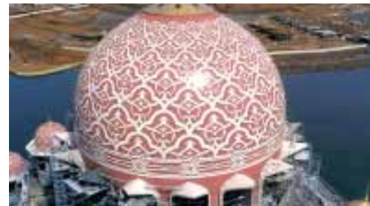
Advanced composites open up new constructive possibilities.
